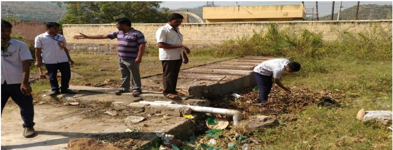
Removing wastage from channel.
