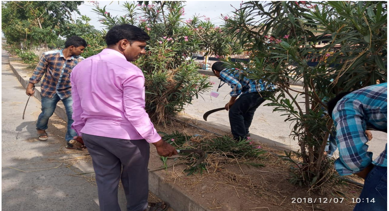
Cleaning on the divider between Gundi – Rayachoty road n 07-12-2018
