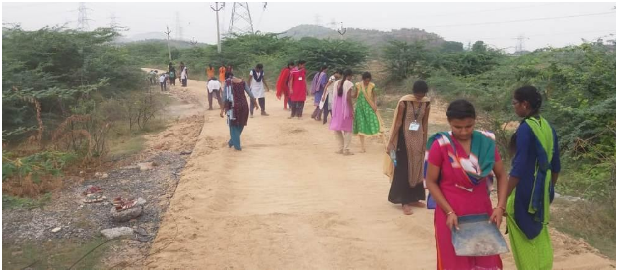
Repairing road from Maruthi to Gundi main road 04-12-2018.
